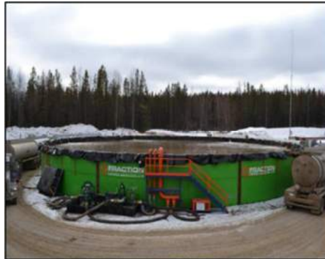
Figure 1.53 Water handling for fracking.
