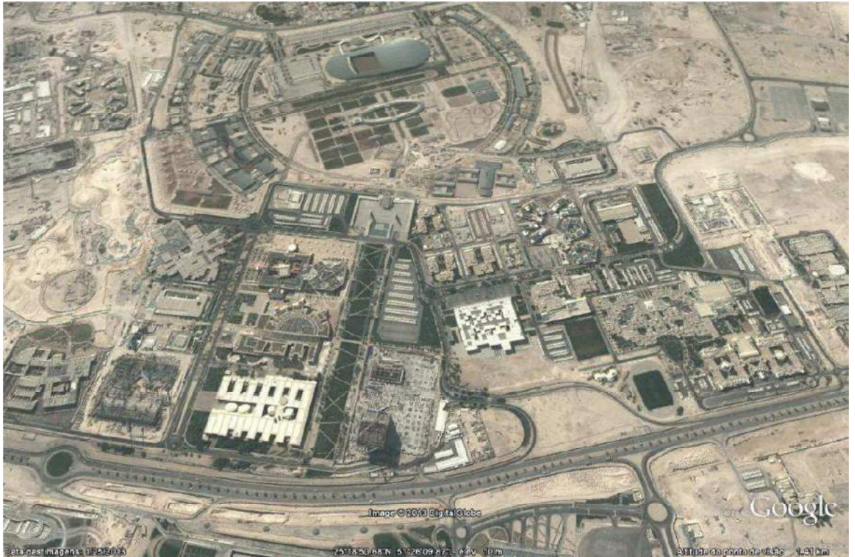
Figure 3.2 When completed, Education City will host 14 km 2 of educational, research, science and community facilities (pictures from http://www.romatreproject.com and Google Earth).
